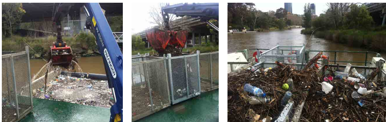
Figure 13 Parks Victoria crane with a bucket grab removing floating litter and debris which is then emptied into wire cages secured to the Pelican vessel
