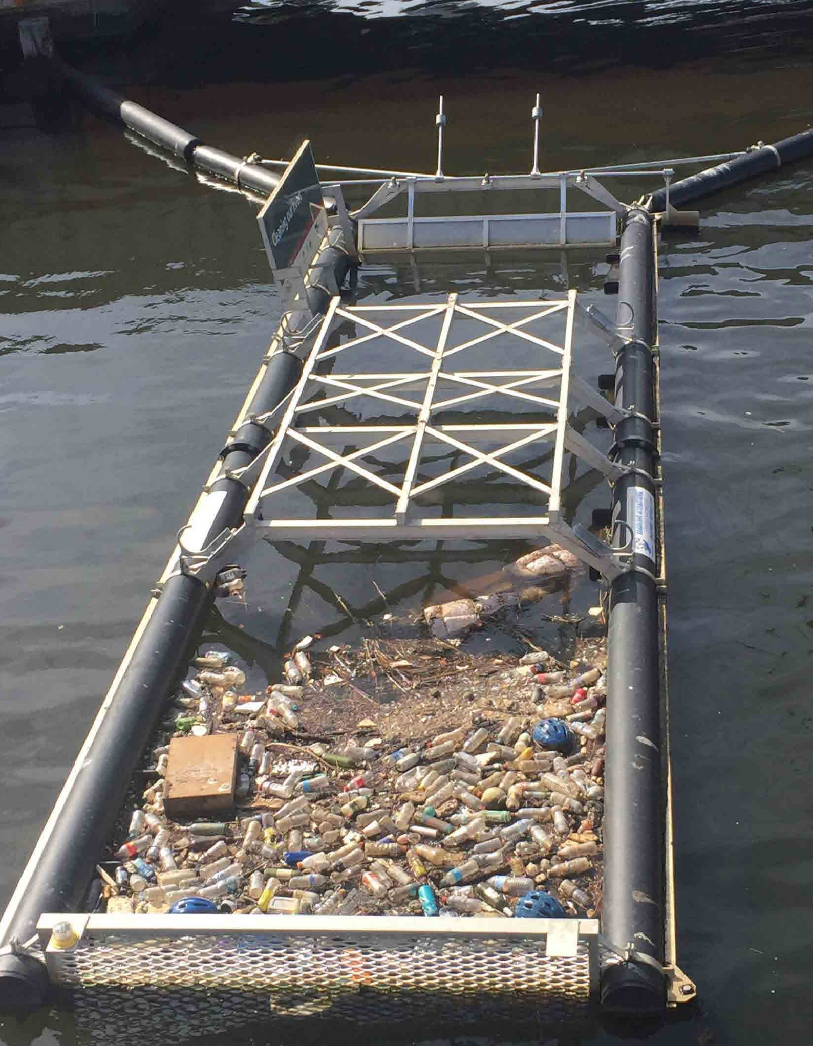
Figure 14 Bandalong litter trap in the lower Yarra River
